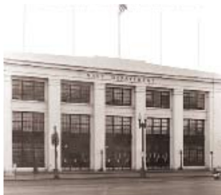
Figura 5. Main Navy Building. Washington D. C. 1953. Cortesía Naval History and Heritage Command.
